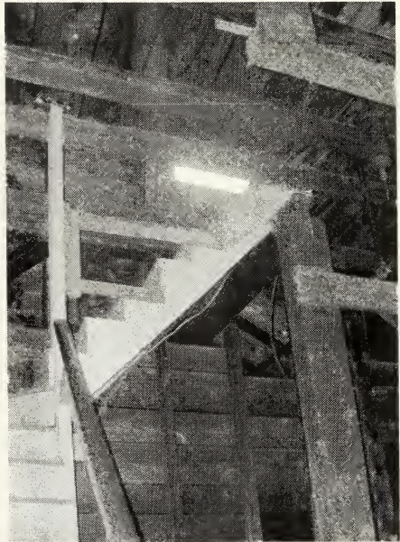
Part of stairway to the clock
